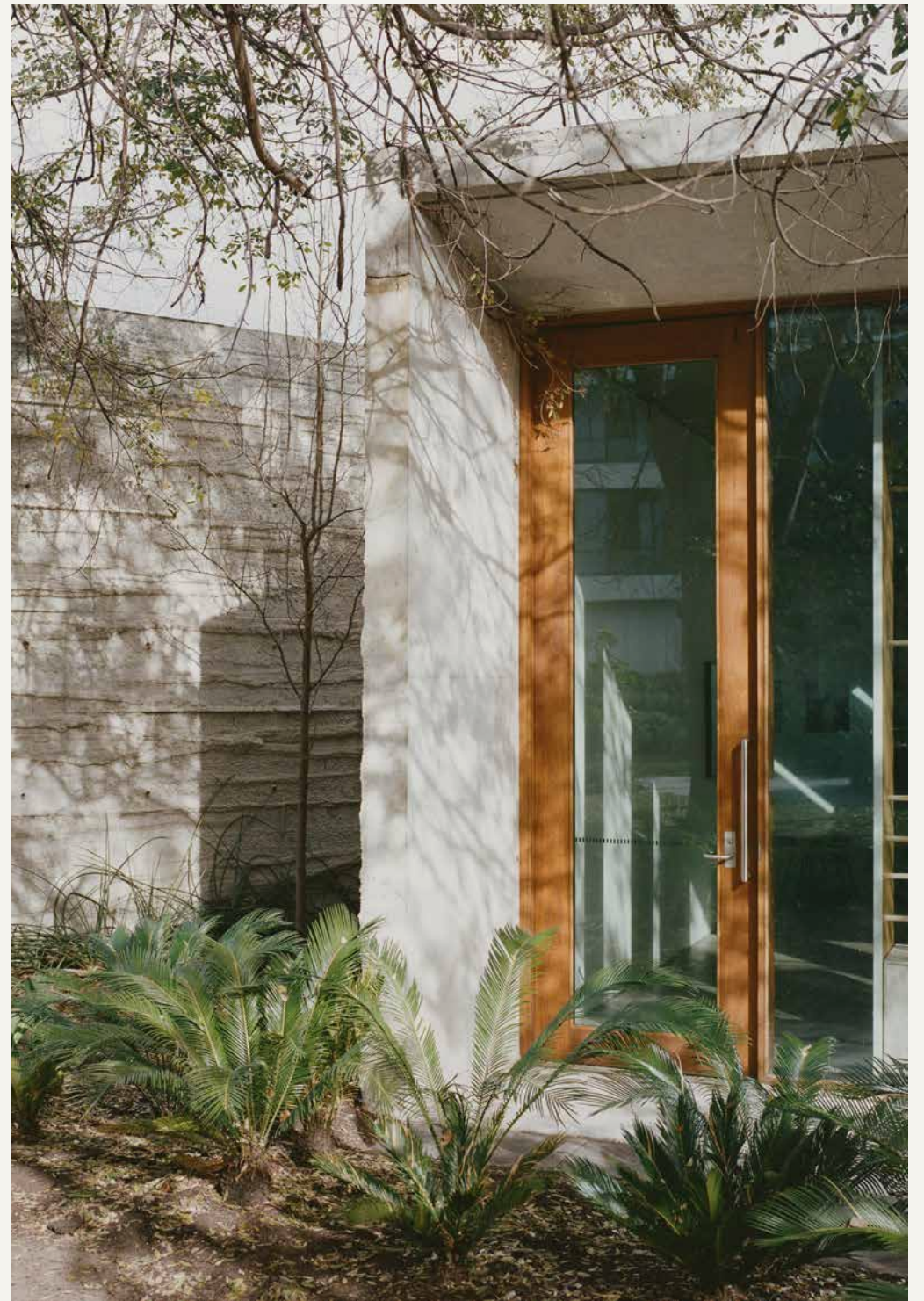
ENTRY, 17 KENDALL LANE
